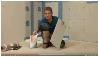
Overboard a floor with 10mm board (video length: 2.5 mins)
