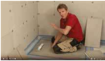
Installing a level access wetroom with a 300mm linear drain (video length: 13 mins)
