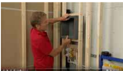
Installing a tileable recessed storage box (video length: 1.5 mins)
